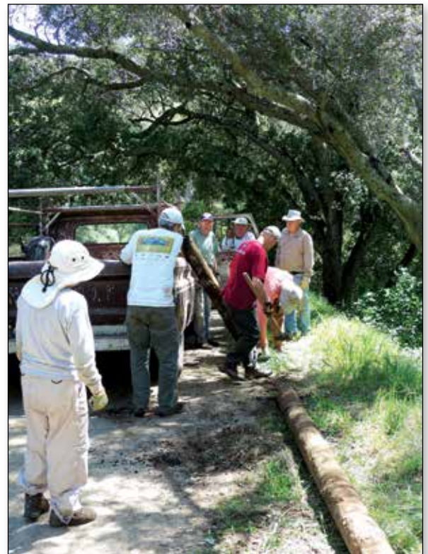
Volunteers remove old water pipes from Sycamore Creek
